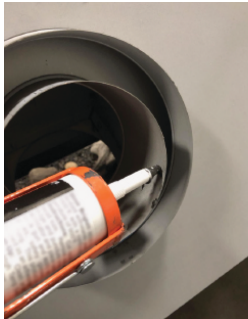
Figure 6.9 - Sealant on Inner Exhaust on Power Vent Assembly
