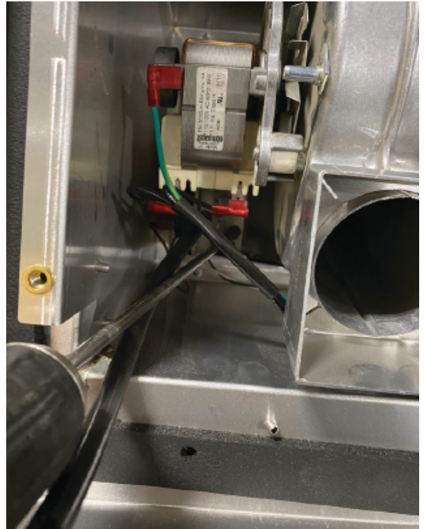
Figure 8.9 - Vacuum Switch Removal
