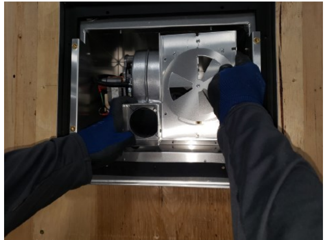
Figure 8.3 - Exhaust Assembly Removal
