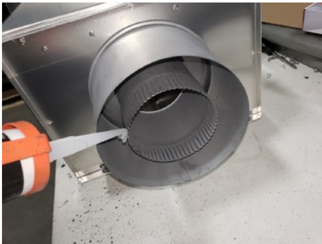
Figure 6.9 - Silicone Inner Exhaust on Power Vent Assembly
