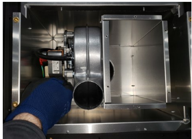
Figure 8.4 - Remove Hot, Neutral, and Ground Wire
