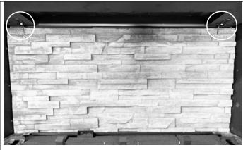
FIGURE 8.3 Back Refractory Panel Installed
