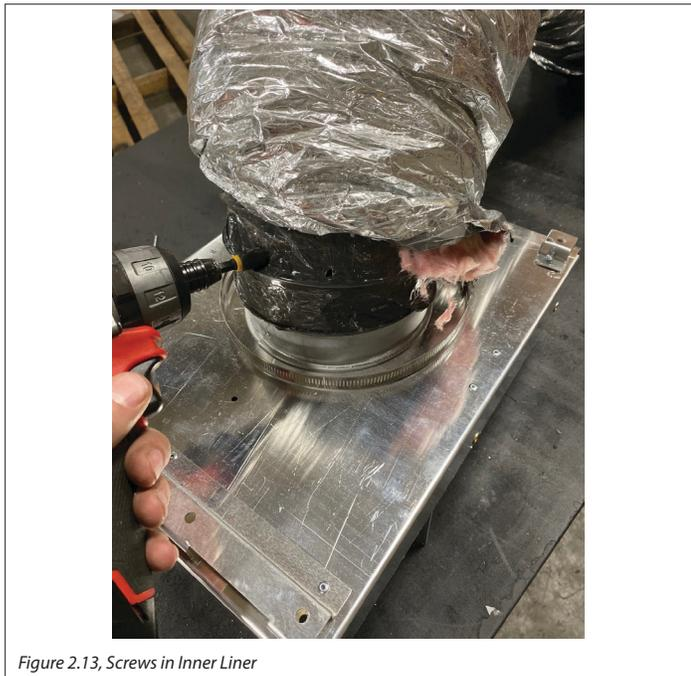
Figure 2.13, Screws in Inner Liner
