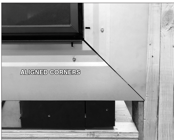
Figure 4.7, Aligned Corners
