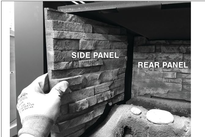
Figure 9.3, Refractory Panel Installation
