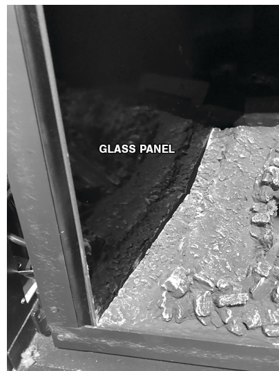
Figure 9.4, Side Backer Plate and Glass Panel Installation
