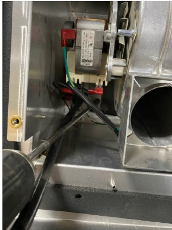
Figure 8.9 - Vacuum Switch Removal
