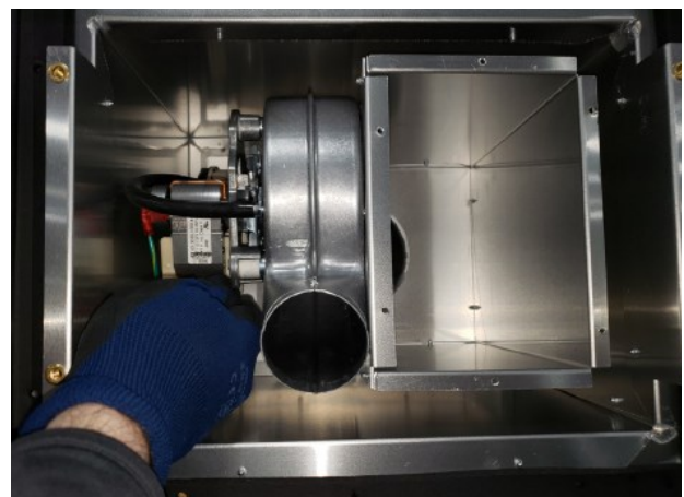
Figure 8.4 - Remove Hot, Neutral, and Ground Wire
