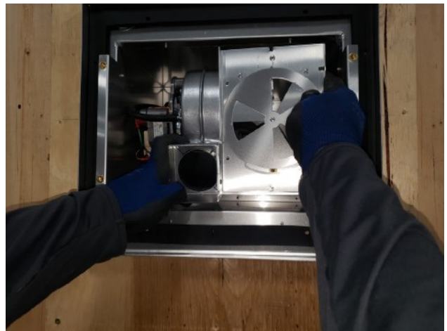
Figure 8.3 - Exhaust Assembly Removal
