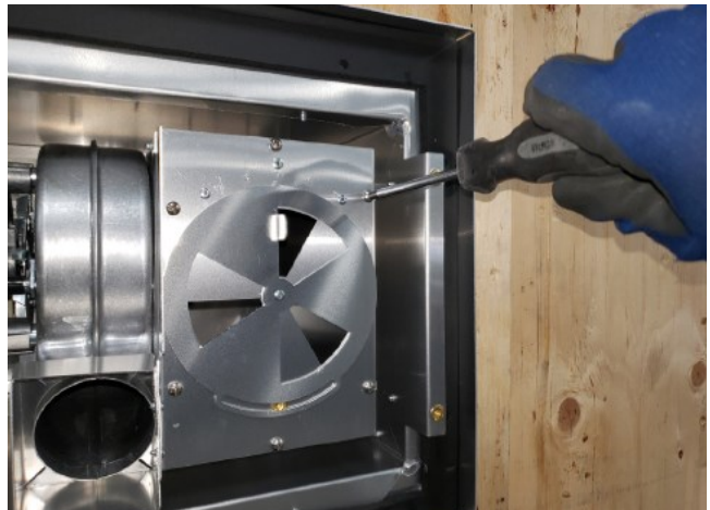
Figure 8.2 - Exhaust Assembly Screws
