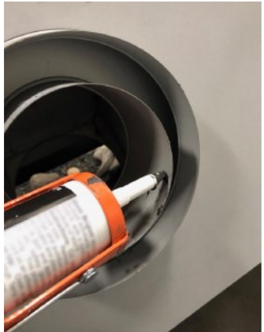
Figure 6.10 - Silicone Inner Exhaust on Fireplace
