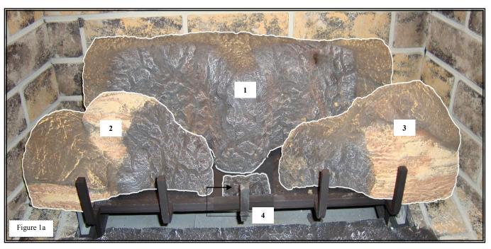
Align holes in bottom of #1-#3 logs with mounting pins on burner, setting down into position. Place #4 log as shown.
