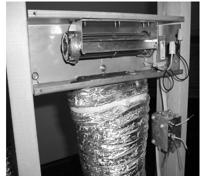
Figure 12.6, Secured Duct Pipe
