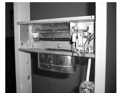
Figure 12.4, Installed Fan Assembly
